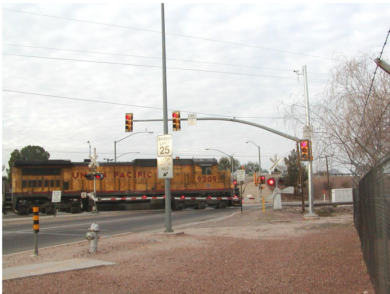
Figure 7: Pre-Signal Installation at Prince Road/UPRR Crossing (12-24-04 Looking West)
